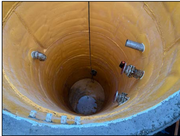
Wet Well after concrete and liner work.
