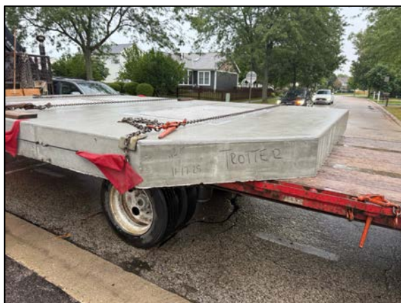
New concrete lid for wet well / valve vault.
