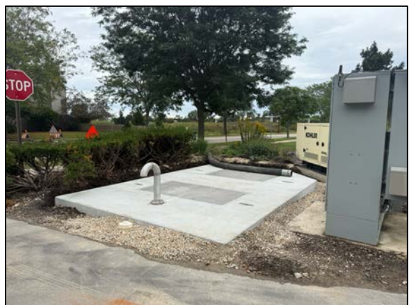
Final install after setting lid.
