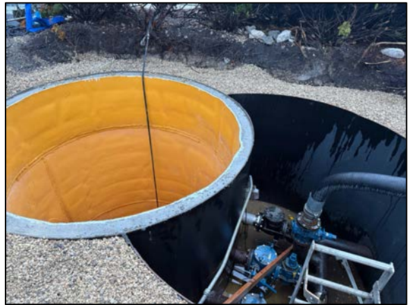
Completed foundation work, prior to lid install.
