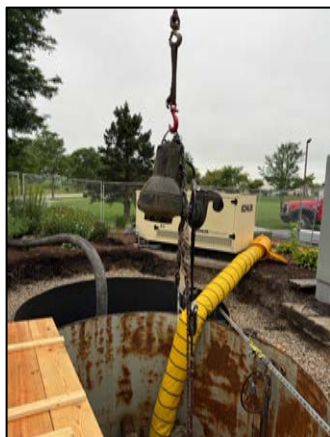
Removal of old pump.
