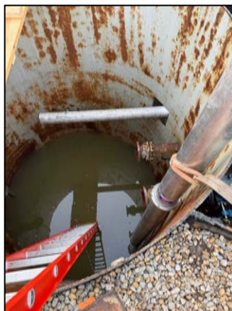
Pipe replacement work.
