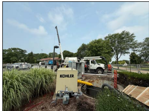
Crane and VAC work for metals removal.
