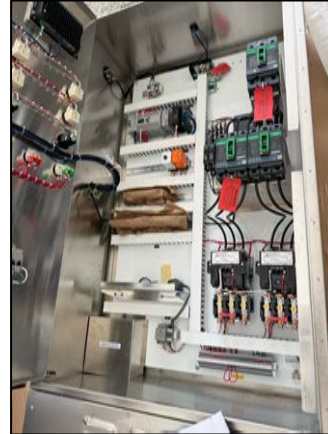
Photo showing new Waterford Panel.
