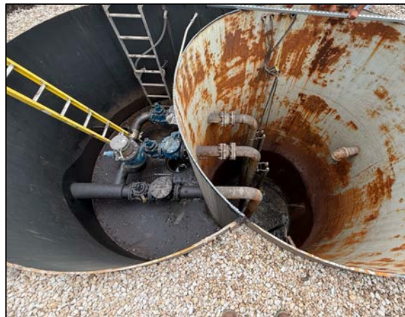
Photo of wet well after lid was cut and removed.
