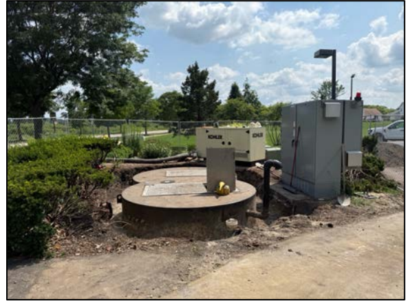
Excavation and concrete lid footing work.
