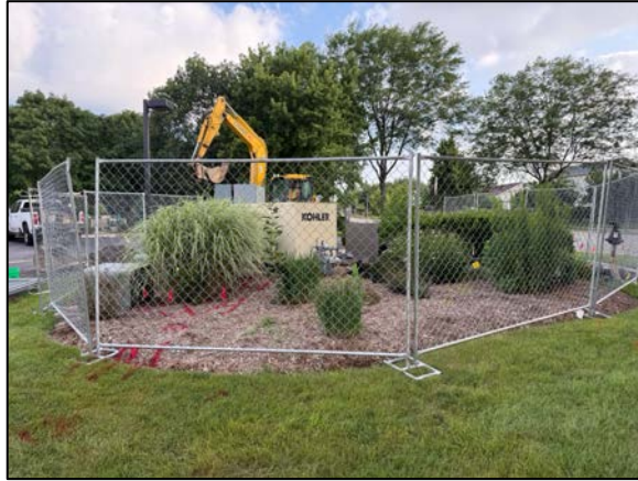
Photo showing project extents.
