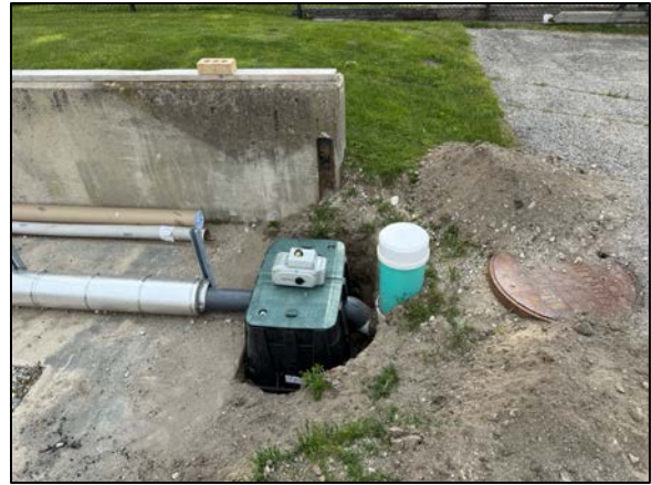
New actuated ball valve install for seepage station.
