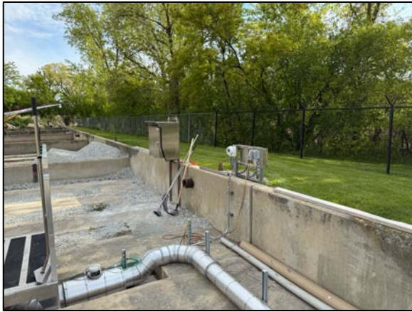
New Elmech Kiosk install for seepage station.
