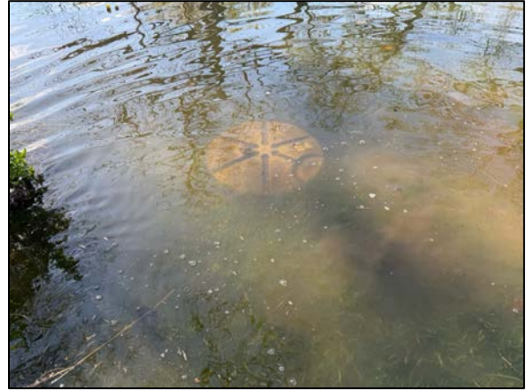
Photo showing fully submerged eOne pit.
