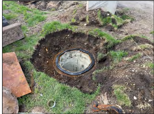
Frame replacement progress during EZ-stik application.
