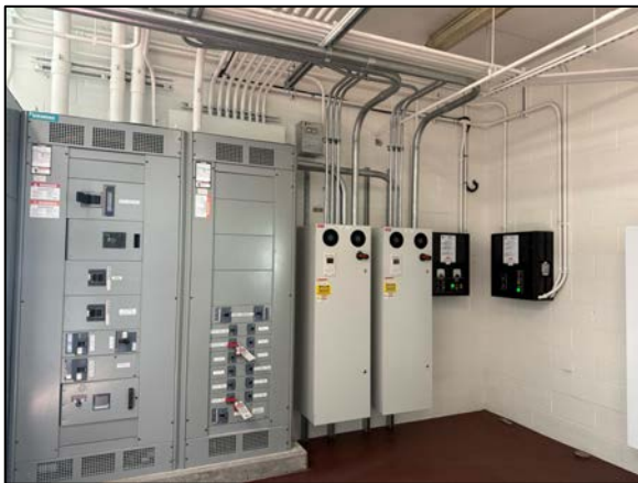
Blower VFD #1 & #2 fully mounted in MCC room.
