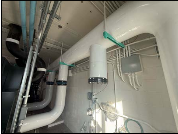
New discharge piping insulation.
