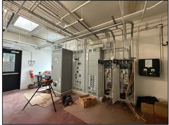
Photo of new ABB VFDs for Kaeser Blowers #1 & #2.
