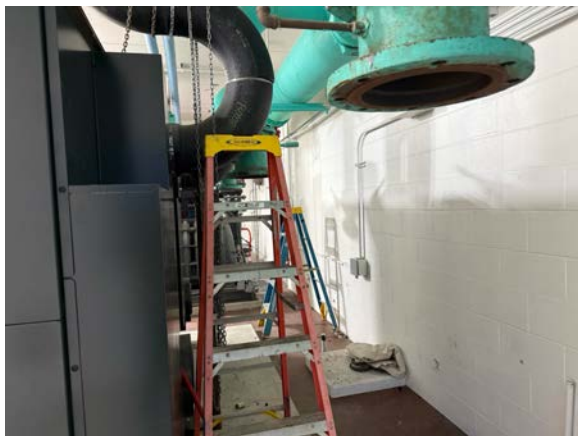
New discharge piping for Kaeser blower #2
