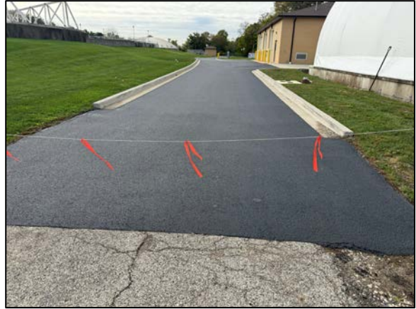
Plant drive after sealcoat.
