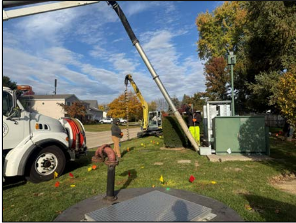
Hydroexcavation assistance for cathodic protection work.
