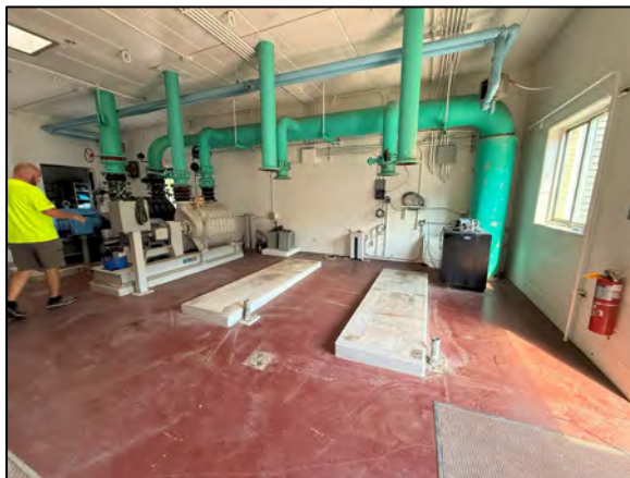
Demolition progress of three (3) Lamson blowers and associated equipment pads.
