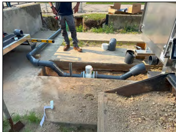
Piping and flowmeter run for septage screener.
