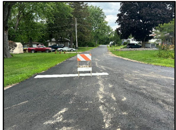
Restored pavement and thermoplastic marking
