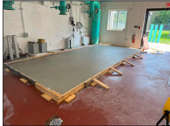
Construction progress of new continuous equipment pad for Kaeser
