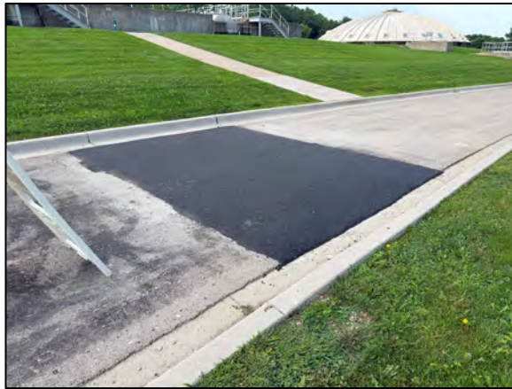
Asphalt repairs for open cut excavation associated with recent forcemain repairs.
