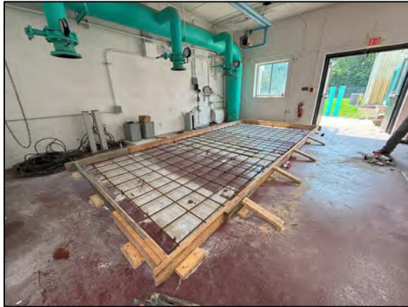
Construction progress of new continuous equipment pad for Kaeser
