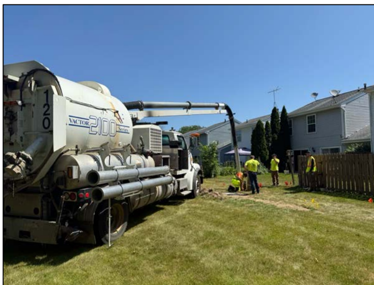
District personnel assisting Bartnick with hydroexcavating for sewer repair work.
