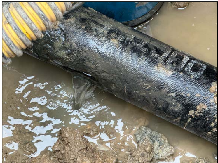
Photo of damaged forcemain.
