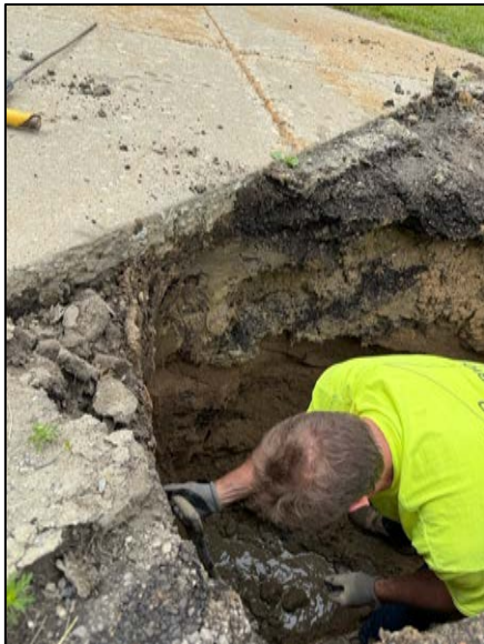
Bartnick excavating for broken forcemain.
