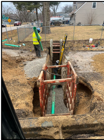
Installation of sanitary services
