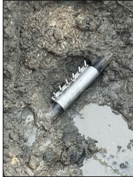
Photos showing the 2" hole and the repair clamp used for the repair.
