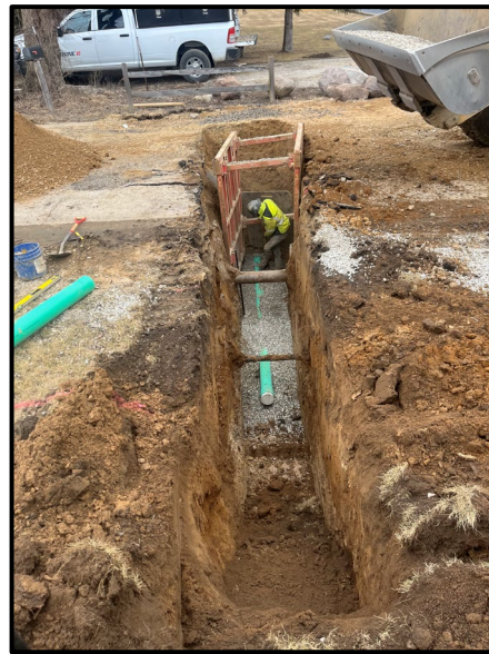
Installation of sanitary services
