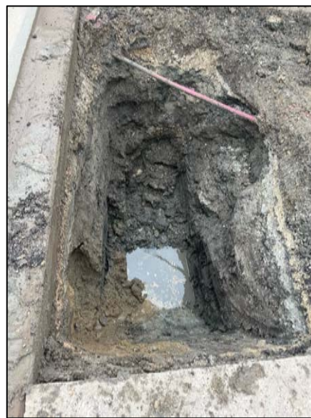
Area of forcemain rupture, under access drive at plant. Excavation progress.
