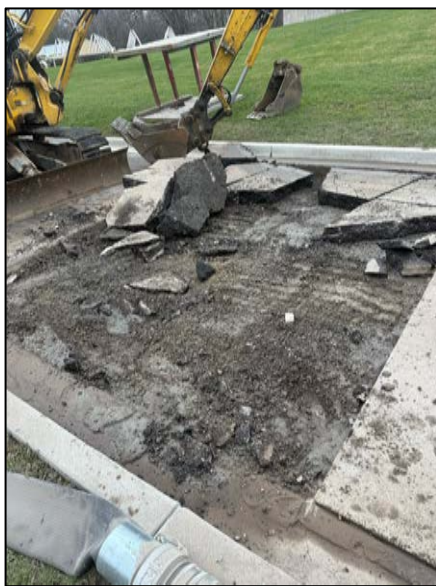
Area of forcemain rupture, under access drive at plant. Excavation progress.
