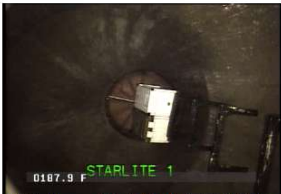
AMH - Access Point - Manhole @ 187.9 ft. END OF SURVEY
