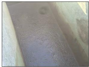
Photo of sludge discovered on bottom of CCT.
