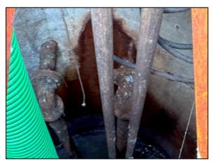
Condition of old wet well metals, heavily corroded.
