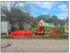
Photo showing station with by-pass pump set-up.
