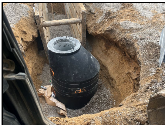
Installation of Manhole 79
