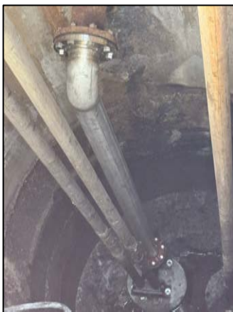
LSS Wet Well Metal Upgrades Includes new base elbows, new stainless steel riser pipes, and new stainless steel upper 90s.
