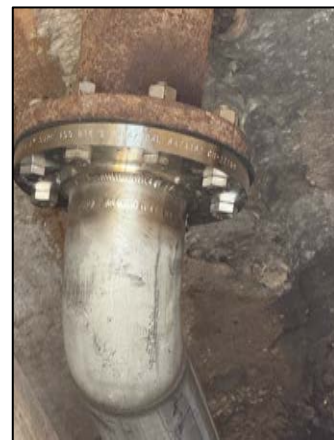
LSS Wet Well Metal Upgrades Includes new base elbows, new stainless steel riser pipes, and new stainless steel upper 90s.
