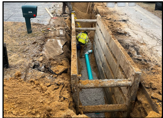
Installed service tee to 2515 Bittersweet Ave
