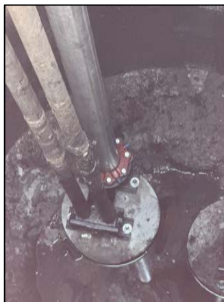
LSS Wet Well Metal Upgrades Includes new base elbows, new stainless steel riser pipes, and new stainless steel upper 90s.
