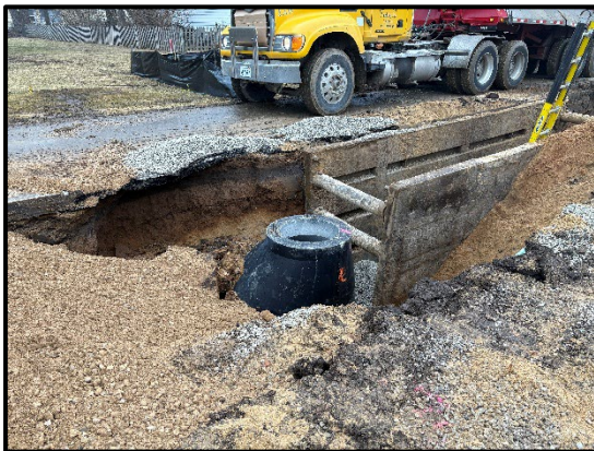
Installation of Manhole 78
