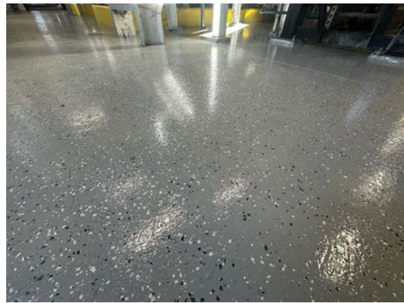
Floor Epoxy in Dewatering Bay.
