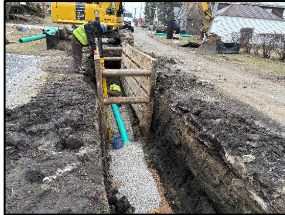
Sanitary sewer main installation on Northeast Shore Dr
