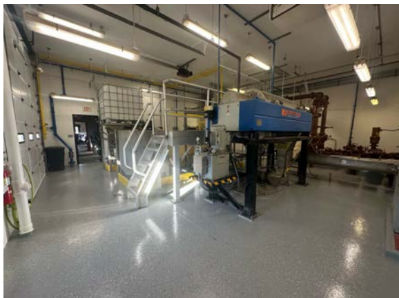
Flooring and Wall/Pipe painting in dewatering bay.
