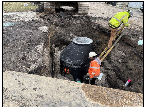
Manhole #63 installation
