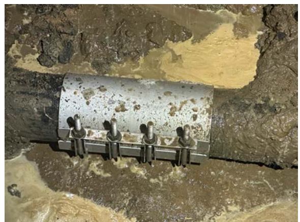
Photo of forcemain after repair
