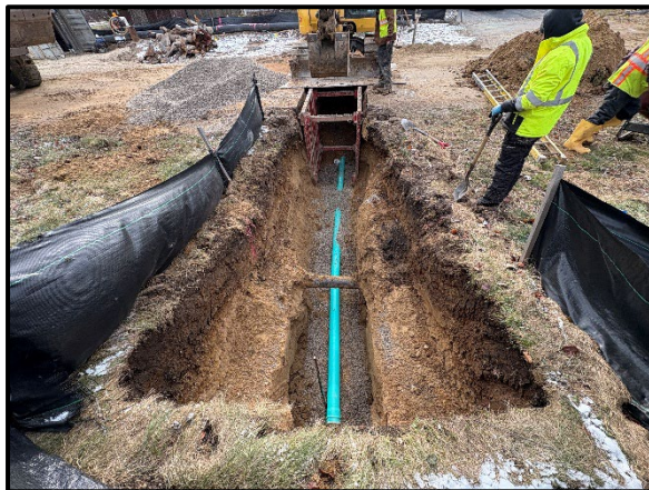
Sanitary service installed at 1510 Pine St
