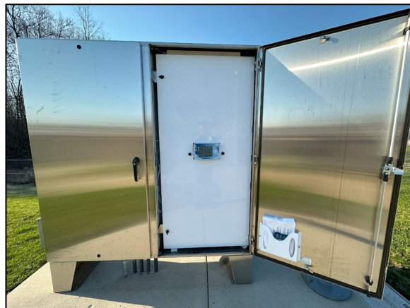
Insite instrumentation transmitter installed at Oxidation Ditch SCADA panel.
