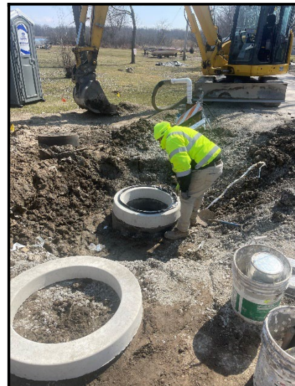
Installation of Manhole Frame
