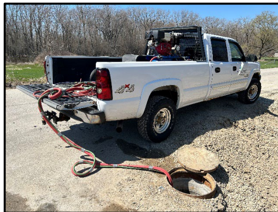
Sanitary Sewer Air Testing
