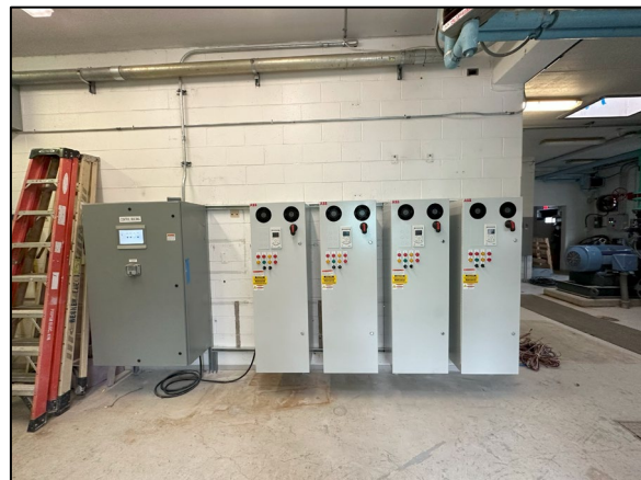
Mounted raw pump VFDs after mini power zone removal.
