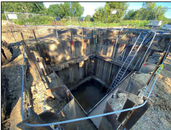
Excavated wet well pit, prior to structure install.
