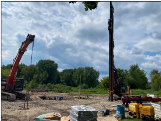
Sheet piles being installed to protect wet well excavation.
