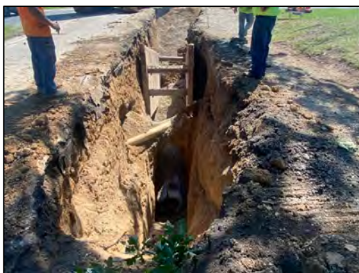
Storm sewer crossing below force main.
