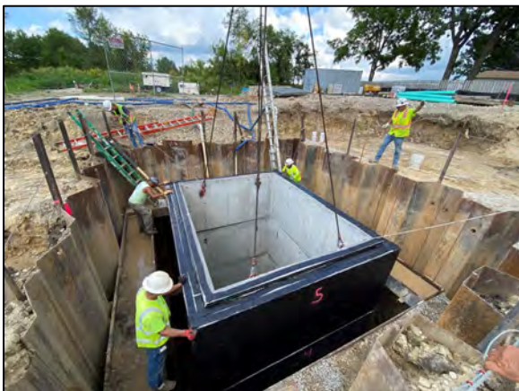
Wet well structure install progress.
