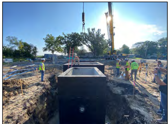
Meter Vault (front) and Valve Vault (back).
