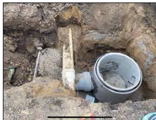
Storm sewer manhole next to force main.
