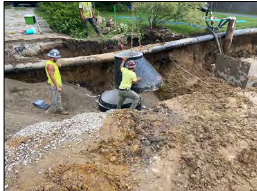
Manhole structure installation at Holiday Hills.
