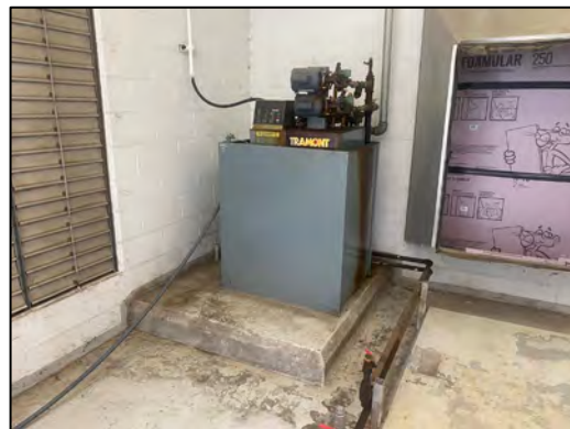
Removal of day-tank is needed for Electrical Upgrades project.
