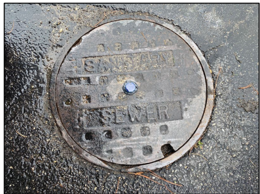
An antenna on top transmits data via satellite.
