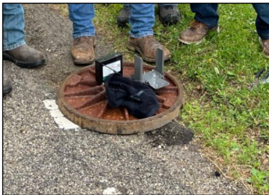
Sensing unit being installed under lid.
