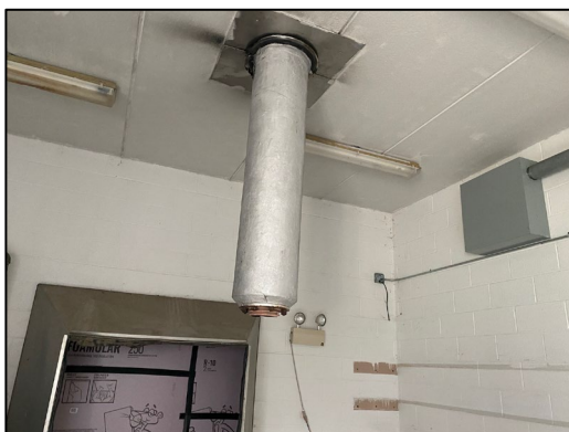
Old generator exhaust pipe may have asbestos insulation.
