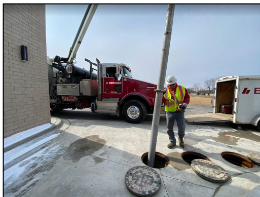
Chipotle Grease Trap being emptied for punchlist inspection.
