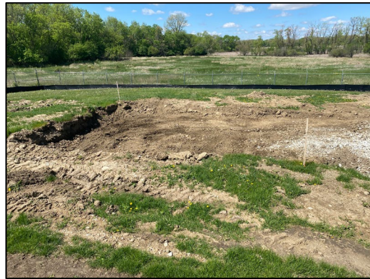
Our skid steer has been quite useful on this project.
