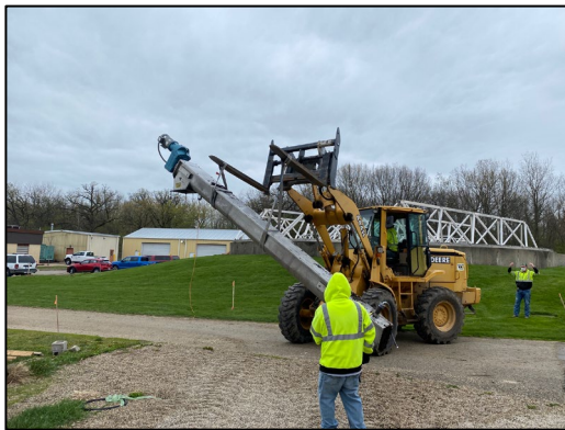
Old sludge conveyor removal.
