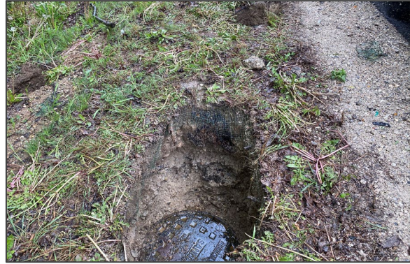
Valve Vault 1. The 2 nd valut was not located due to road undermining concerns.
