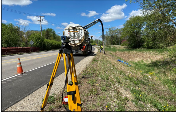
Hydroexcavating with District Vac and surveying equipment.
