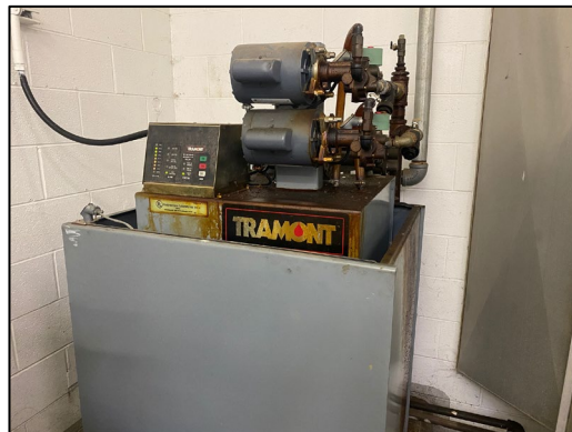
The day tank is equipped with pumps to draw from the bulk tank.
