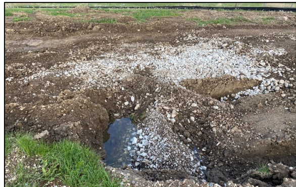
Water pooling at sub-grade. Stone is being added to allow for steer to move.
