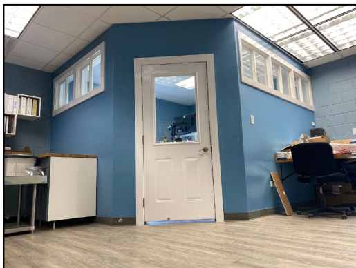
Completed walls with windows to allow light to pass through.
