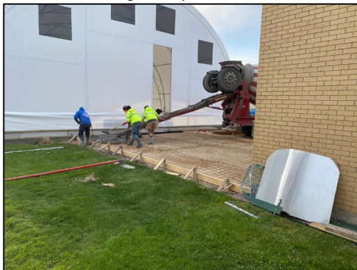
Concrete pad being poured.
