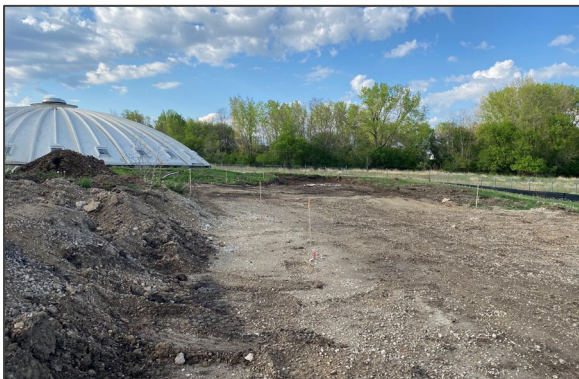
Excavated area utilizing District skid Steer and surveying equipment.
