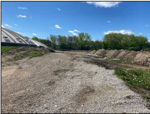
Gravel driveway was widened to allow work on the North Clarifier.
