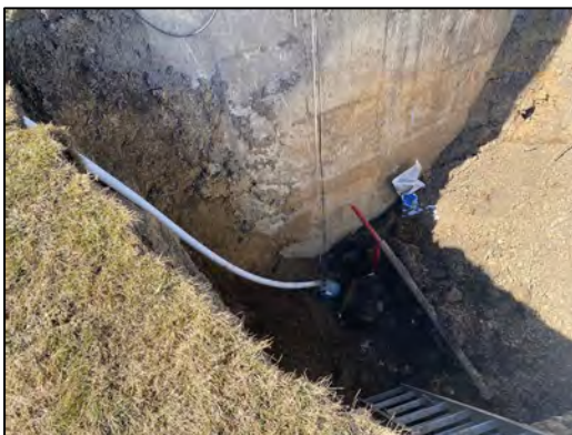
Drain valve excavation.
