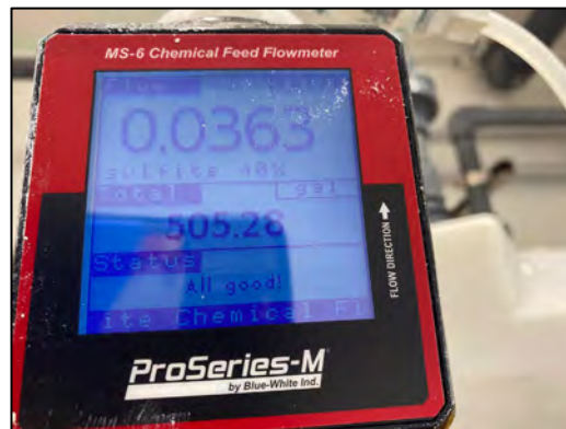
Sodium Bisulfite Flowmeter.
