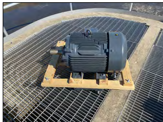
New motor awaiting installation.
