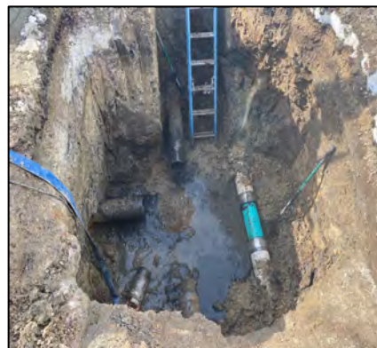
Sludge line excavation.
