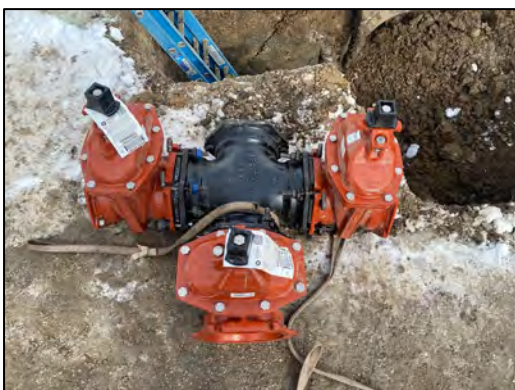
Sludge Cleanout assembly.
