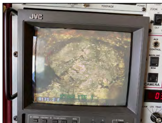
Televising camera’s view of heavy grease as service connection.
