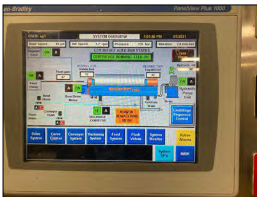
Centrifuge control panel in Dewatering Building.
