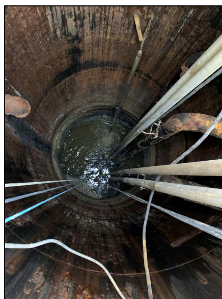
LS6 – 2 weeks after grease trap cleaning.
