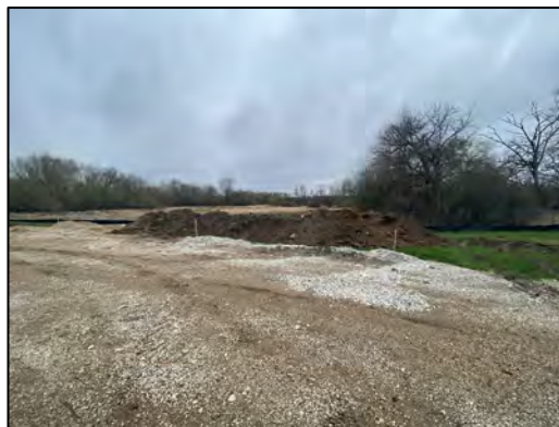
Spoils piles were consolidated into one pile.
