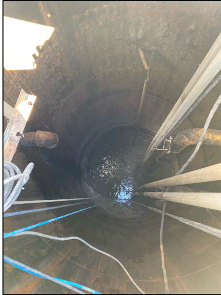
LS6 – 3 weeks after grease trap cleaning
