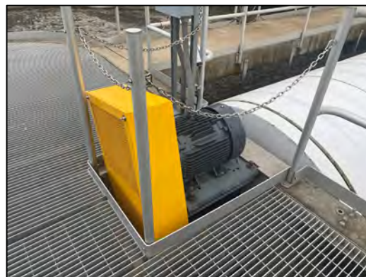
New motor and freshly coated belt guard.
