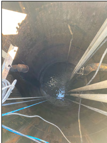
LS6 – 5 weeks after grease trap cleaning.
