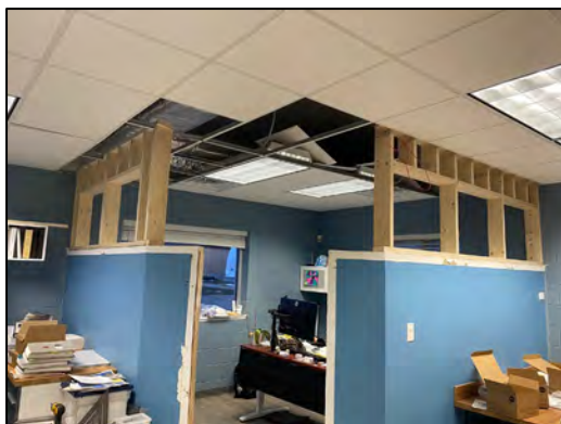
Initial framing of the wall extensions.
