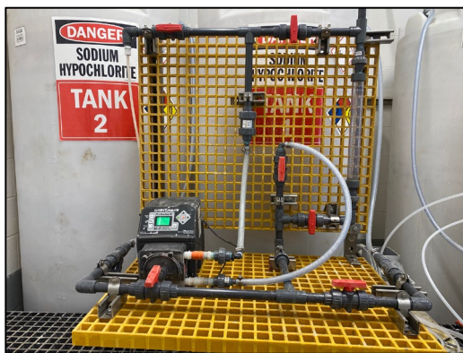
Our new homemade chemical feed skid.
