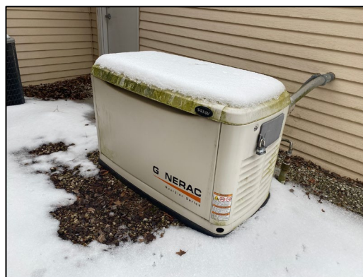
The District Office generator has seen better days.
