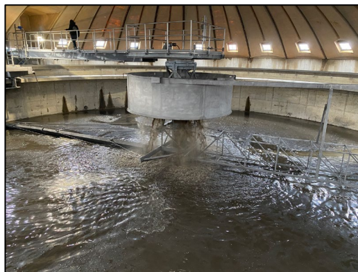
Filling of the North Clarifier.
