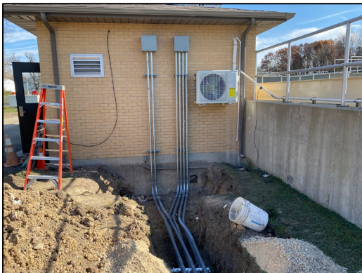
New conduits leaving Chemical Building.
