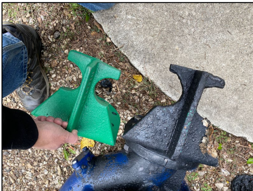
Replacement flange compared to old.
