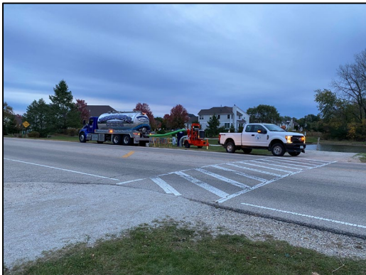
Bypass pumping staging area.
