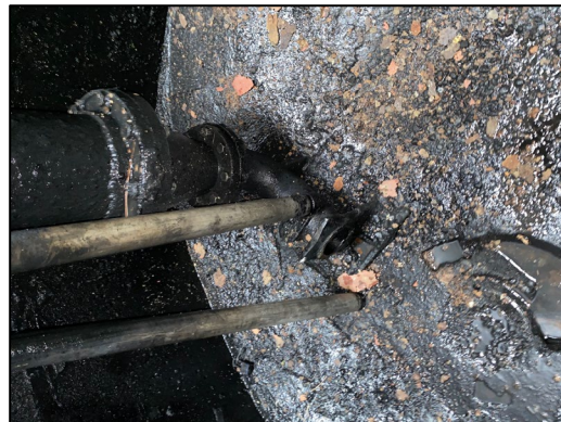
Base elbow and separated guide rail.
