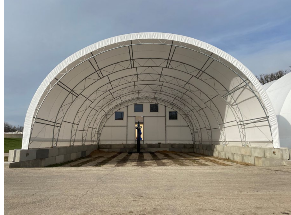
Picture of inside of the new sludge drying bed cover.
