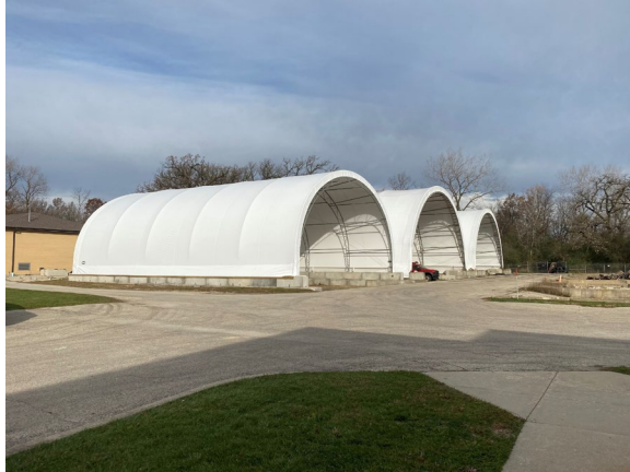
Picture of new sludge drying bed cover.
