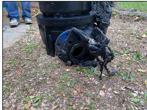
Extremely loose flange on pump.
