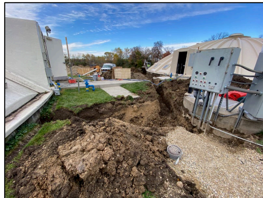
Trenching for conduit bank installation.
