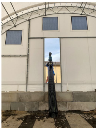
Picture of the endwall opening for conveyor penetration.
