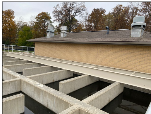
Bridge placed and awaiting grating and rails.
