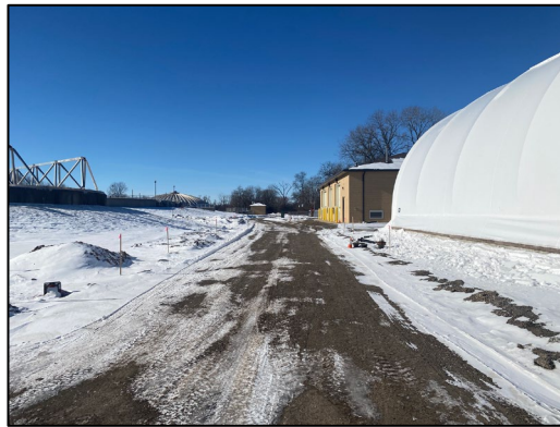
Curbs removed and stone graded.
