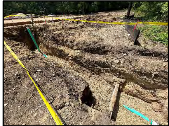
Newly Installed Sanitary Sewer Connection to Existing Manhole
