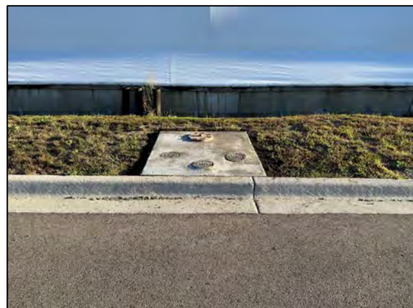
New concrete slab surrounding b-boxes and flange.
