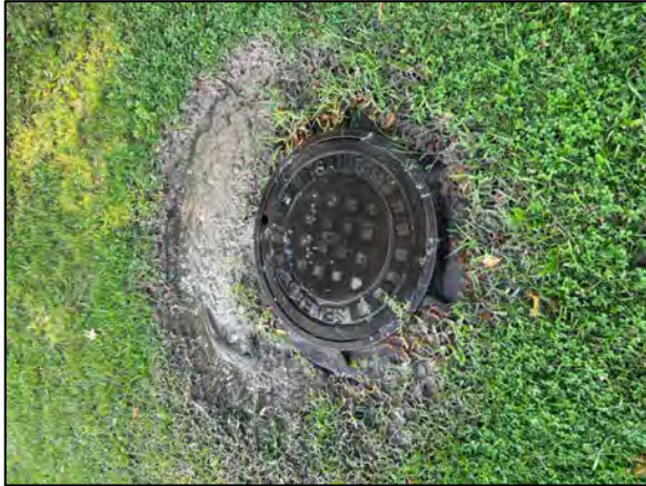
MH B8SE14 (1 of 3 manholes that surcharged).
