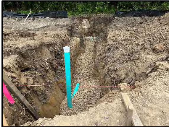
Newly Installed Sanitary Sewer Connection to Existing Manhole
