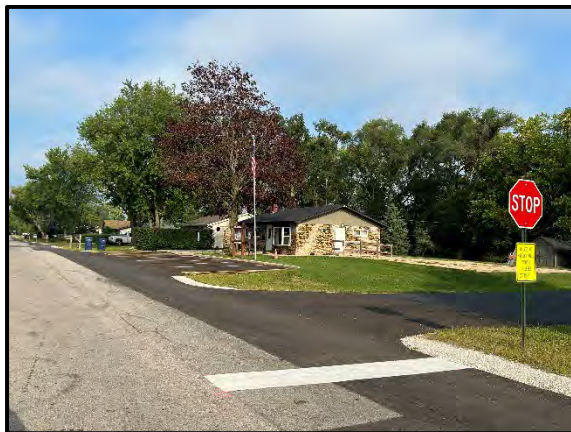
Thermoplastic Pavement Marking at Holiday Hills Village Hall
