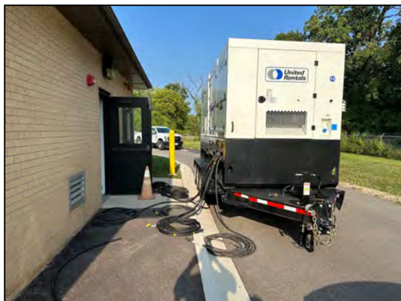
Chemical equipment temp power from backup Generator.
