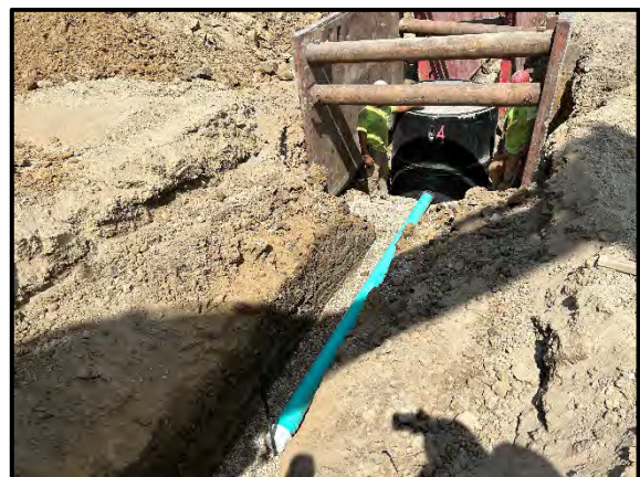
Installation of New Manhole and Sewer
