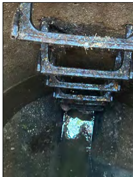
Photo of MH C8NW31 after roots removed.
