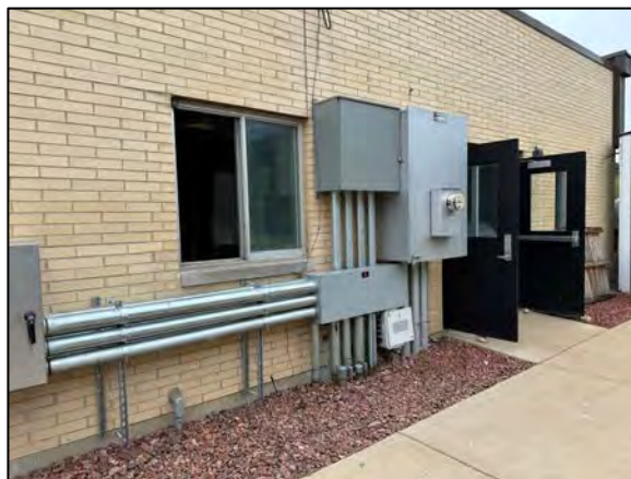
New exterior junction box located above floodplain.
