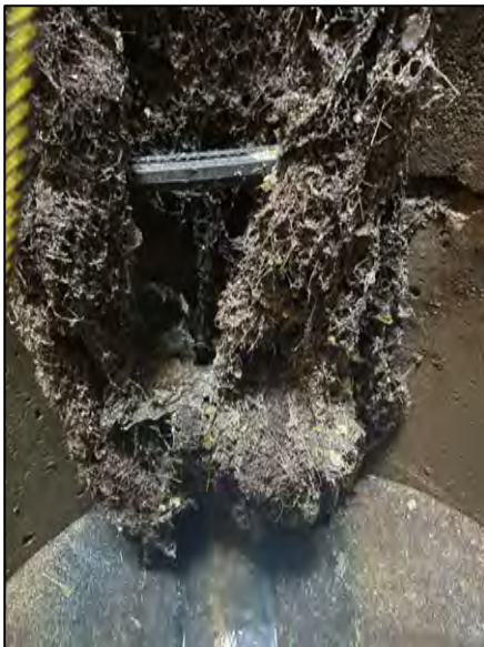
Root intrusion blockage found within MH C8NW31.
