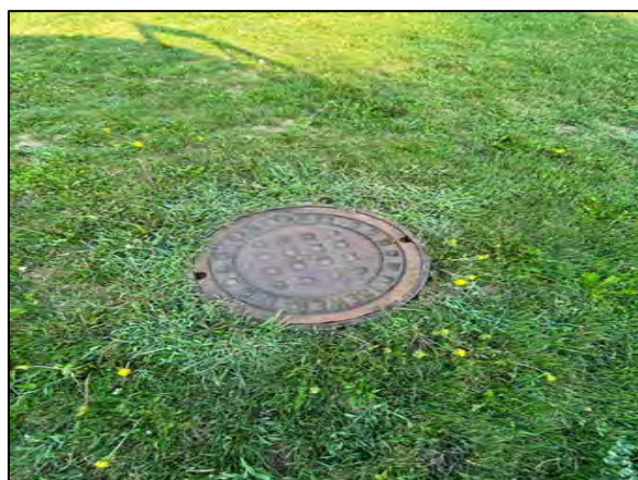
MH B8SE14 (1 of 3 manholes that surcharged).
