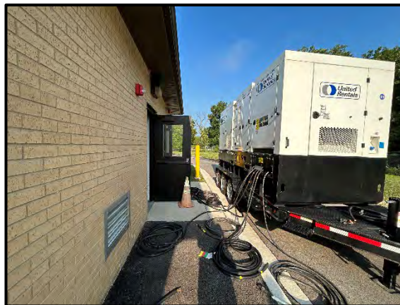
Backup Generator for Chemical Equipment
