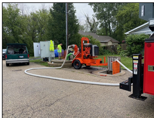
Bypass pump being set up at Lift Station 5
