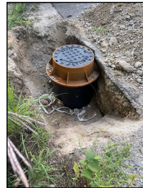
VV1 raised to grade, avoiding damage to road shoulder.
