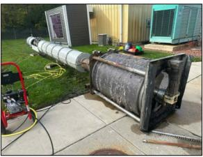
RDS unit after pulled out of Headworks.
