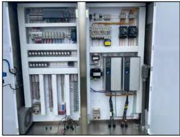
Low and high voltage components separated for safety.
