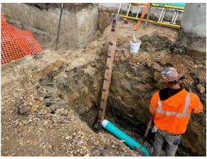
Pipe plugged & marked for plumbing connection.
