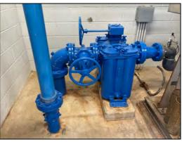
This strainer filters treated water for reuse in our facility.
