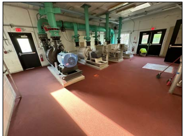
Flooring progress after grit coat.
