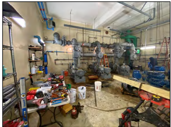
Basement valve/pump work progress during bypass.
