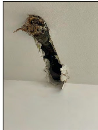
Branch Punctured through Roof and Ceiling
