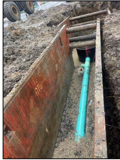
Sanatory Sewer Installation on Hickory St.
