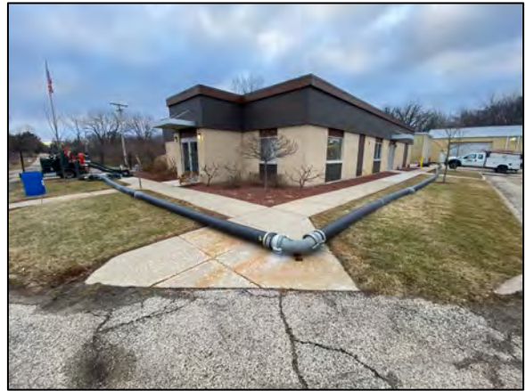
Bypass pipe routing around Control Building.
