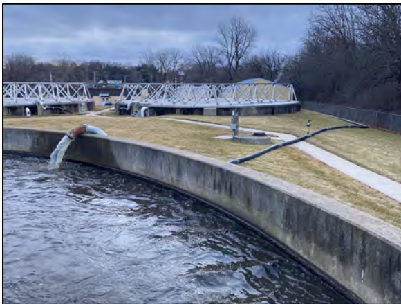
Bypass discharge location into Oxidation Ditch.
