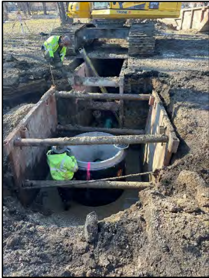
Manhole #41 Installation on Hickory St.
