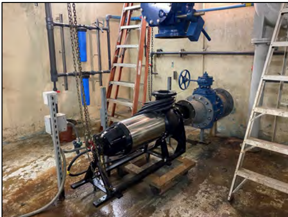
New submersible Grundfos Raw Pump #1.
