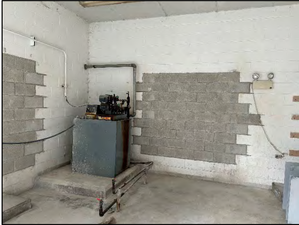
Current standing after CMU block installation.
