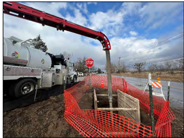
Dewatering for force main install on River Road.
