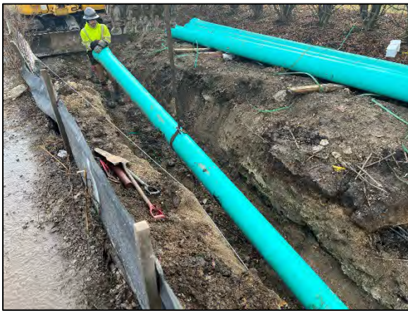
Force main installation on River Road.
