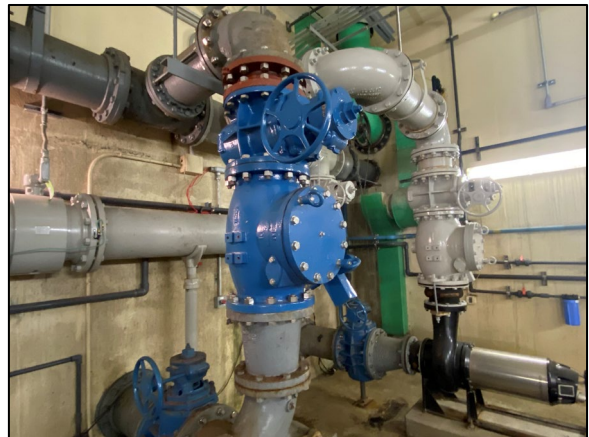
New valving for all raw pumps. This shows Raw Pump #3.
