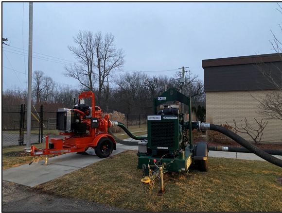
Two bypass pumps used for bypass event.
