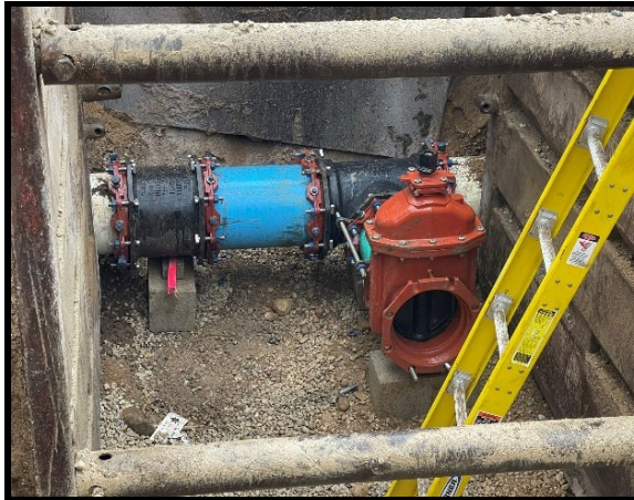
Connection to existing Force main on Lily Lake Rd
