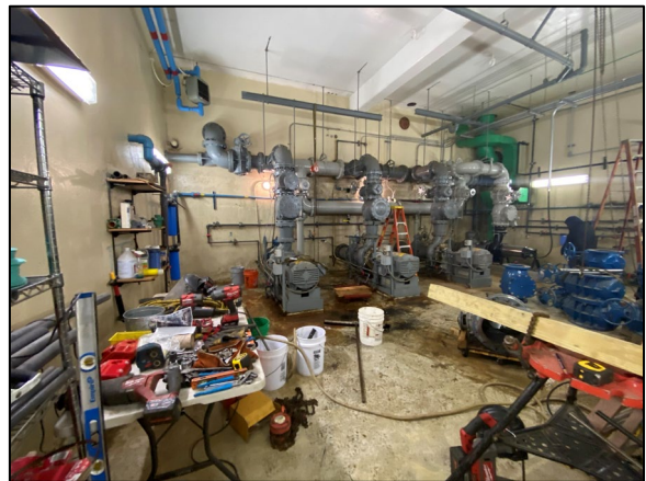
Basement valve/pump work progress during bypass.
