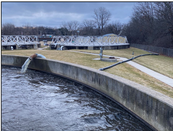
Bypass discharge location into Oxidation Ditch.
