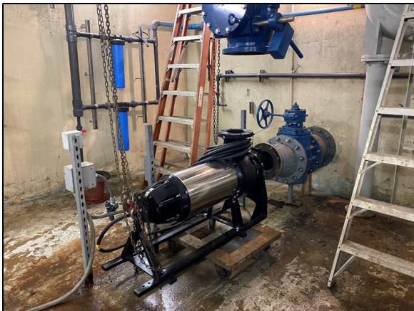
New submersible Grundfos Raw Pump #1.
