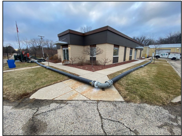
Bypass pipe routing around Control Building.
