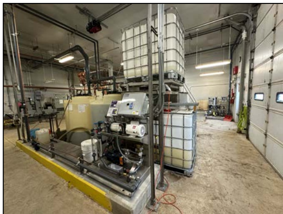
Photos showing new Polymer Skid and Tote Tilter Setup for Dewatering.
