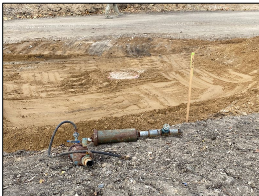
Old cast iron air release valves.
