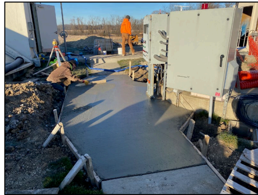
New concrete pad poured to support new panel.
