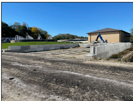
Fully constructed block foundation.
