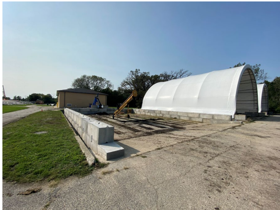
Picture of completed block foundation.
