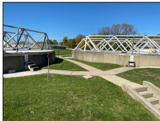
New pads at access hatches on digesters.
