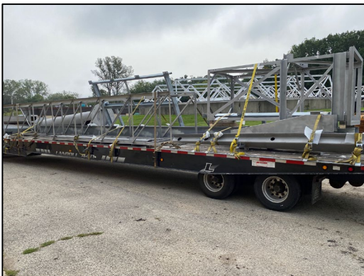
North Clarifier mechanism being delivered.
