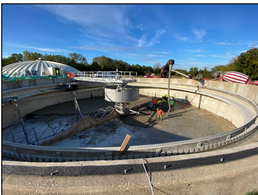
Floor grout being poured.
