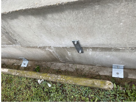
Picture of strapping installed on block foundation.
