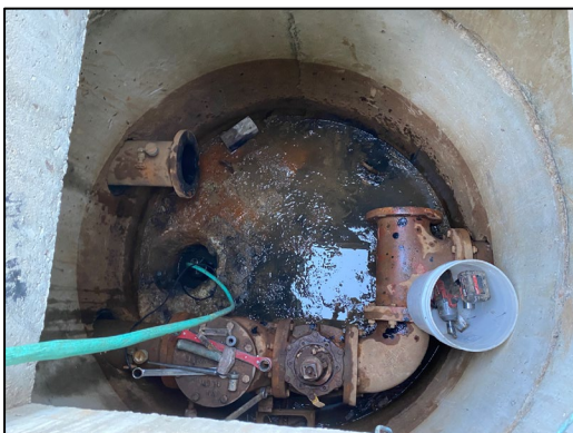
Dry well with one old assembly removed.
