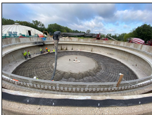
Pouring process and finished concrete floor slab.
