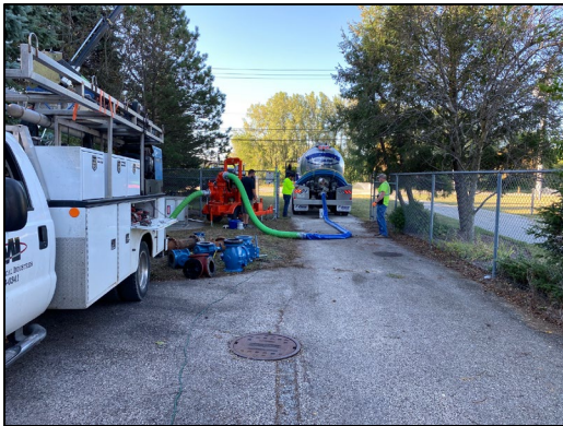
Bypass pump connected to septic tanker.
