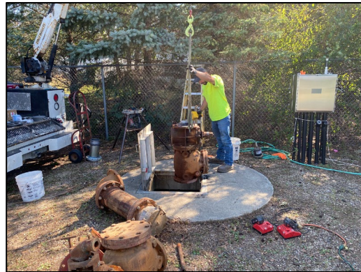
Old isolation and check valve assembly.
