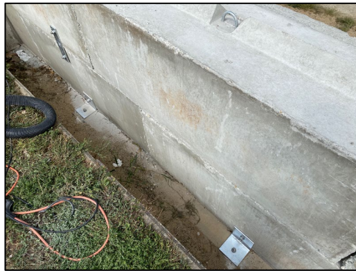
Anchors and straps installed.
