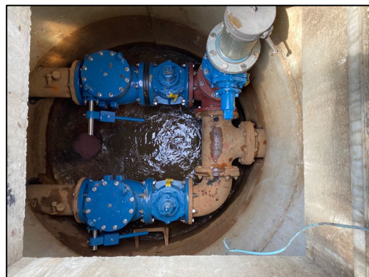
New isolation and check valve assemblies with bypass port.
