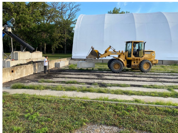
District employees transferring and placing block foundation.
