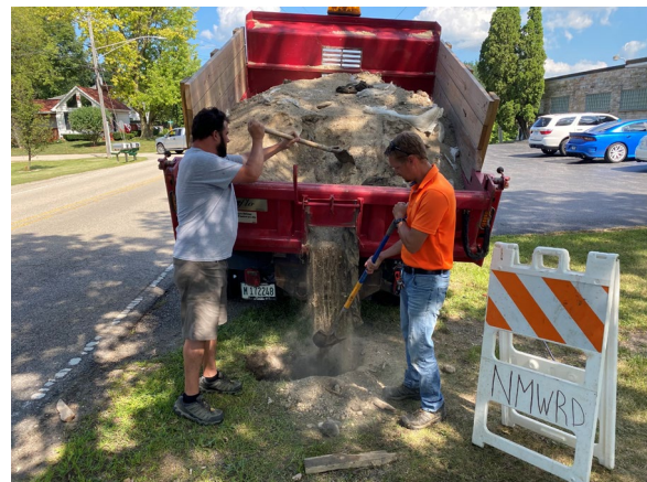
Backfilling exploratory pit.
