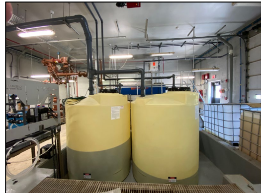
Bulk tanks with supply and feed lines.
