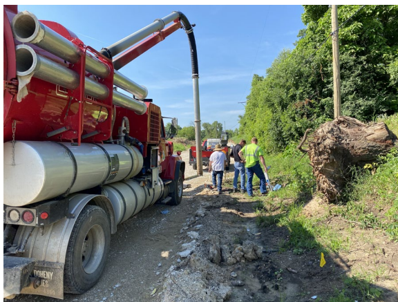
Picture of hydro excavating for 12" forcemain at Lily Lake Road.
