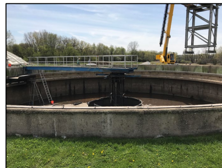
A progression of the dome removal and demolition of the interior mechanisms.
