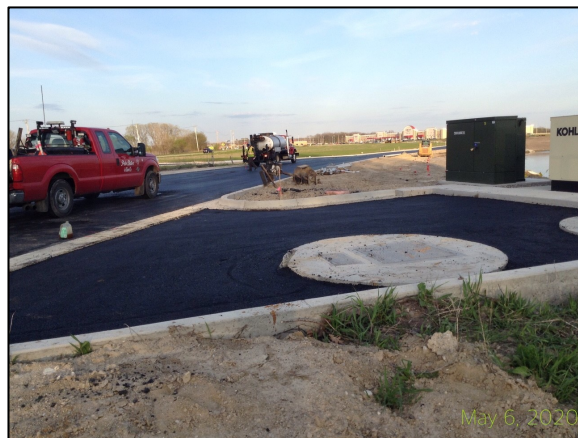
Figure 1. Woodman's Lift Station with roadway base course pictured.
