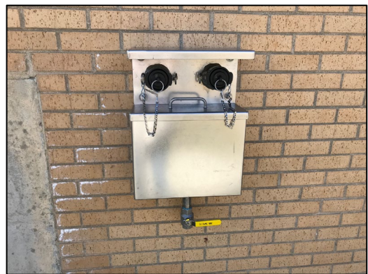
Exterior fill ports with spill containment reservoir
