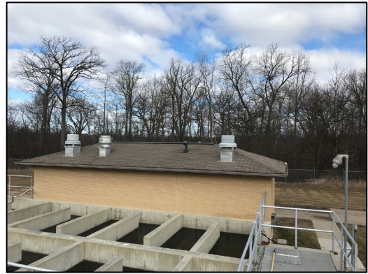
Rooftop venting will reduce interior vapors
