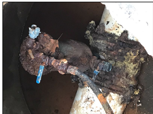
Heavily corroded air relief valve
