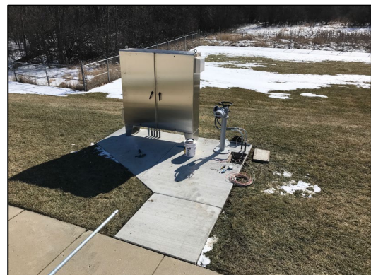
Oxidation Ditch SCADA panel
