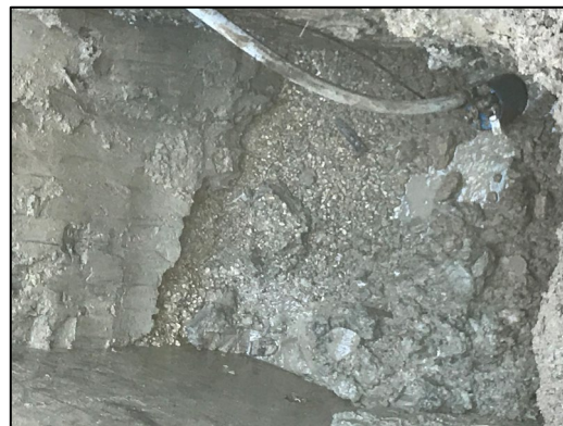
Picture of PRV bedding.
