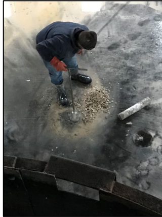
SRN team hand augering for soil boring.
