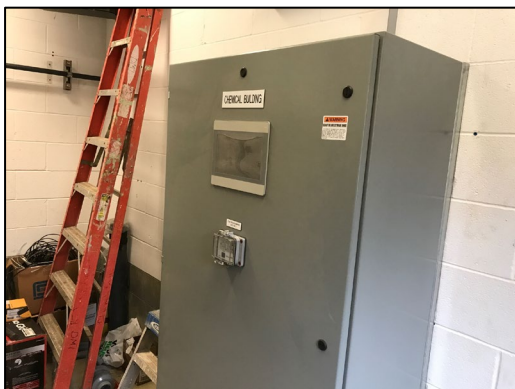
Chemical Building SCADA panel
