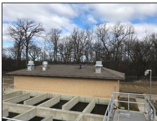
Rooftop venting will reduce interior vapors
