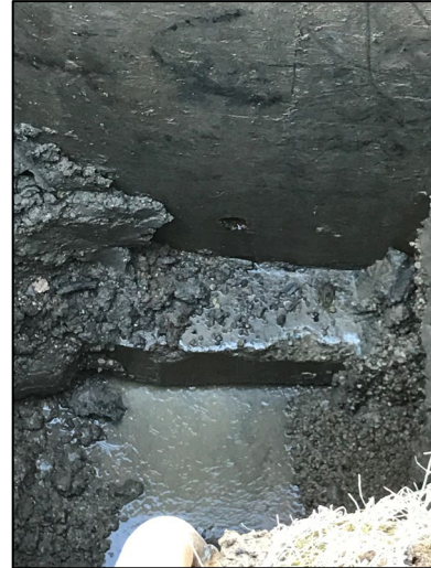
Picture showing extent of Clarifier footing.
