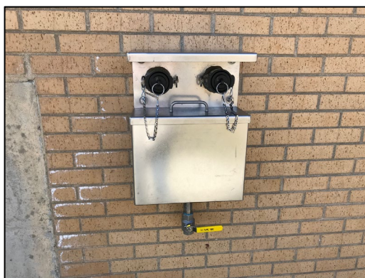
Exterior fill ports with spill containment reservoir
