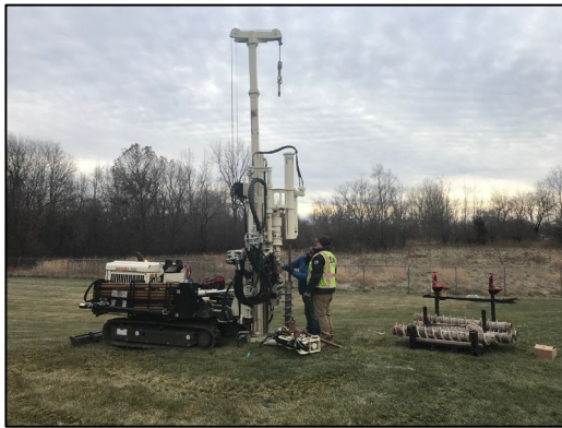
Monitoring well installation and boring collection.
