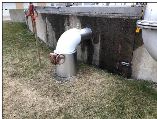
New heat trace and insulating wrap.
