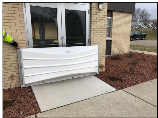
Fiberglass flood stoplog.
