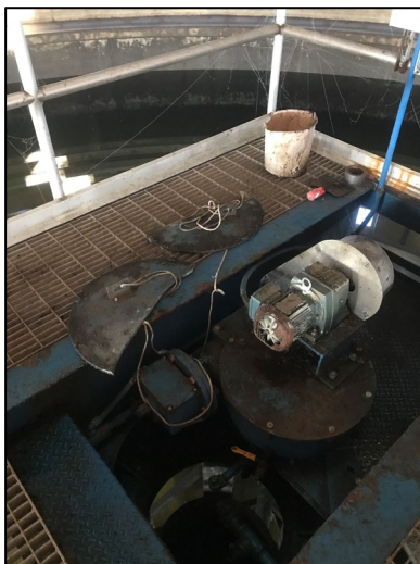
Feedpipe "cover" after cut was made.
