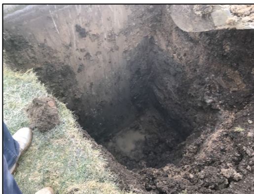
Digging down to inspect the pressure relief valves.
