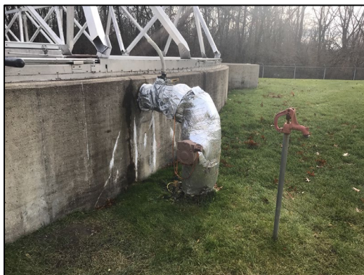
Preexisting insulation and heat trace.
