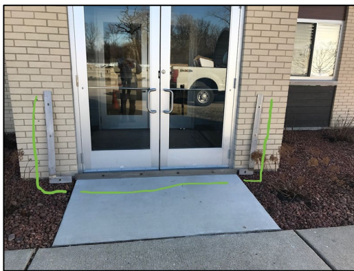
Metal mounting and sealing plates.
