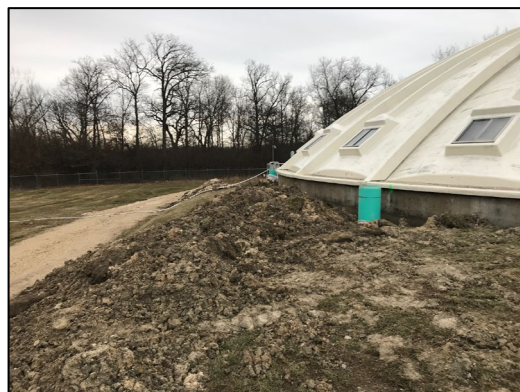
Stand-pipes installed after excavations.
