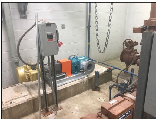
New Sludge Pump prior to install last summer.
