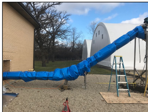
Heat trace cable and an insulating wrap to protect against freezing.
