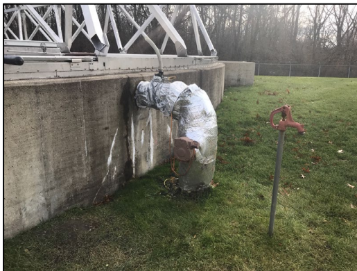
Existing insulation and heat trace.
