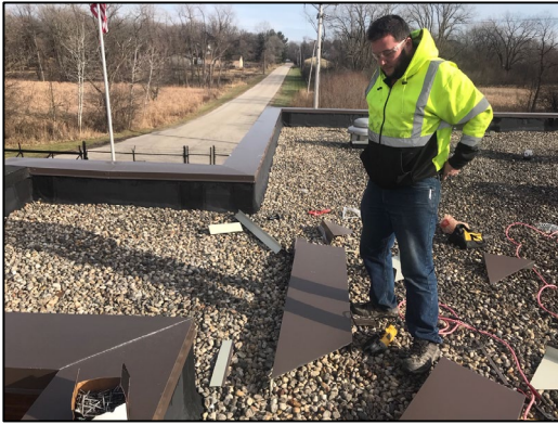
New coping installed on top of perimeter wall.
