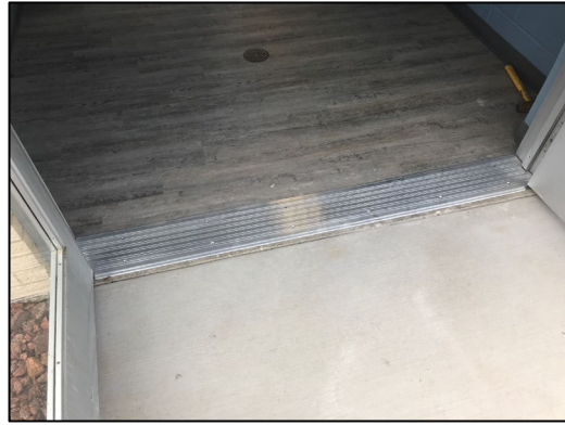
New thresholds installed at exterior doors.
