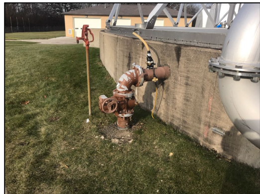
Piping being prepped for new freeze protection.
