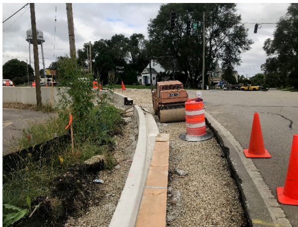
Picture of newly poured curb for right-turn lane.
