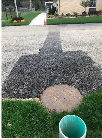
Picture of new manhole for septage receiving.
