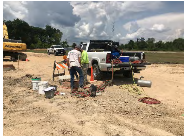
Picture of manhole vacuum test.
