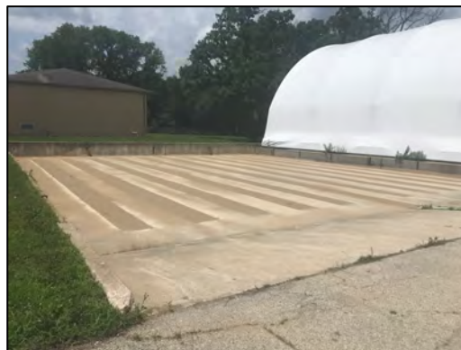
Ready for a roof, and some sludge!
