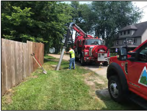
Hydro-excavation to reach break in low pressure force main.
