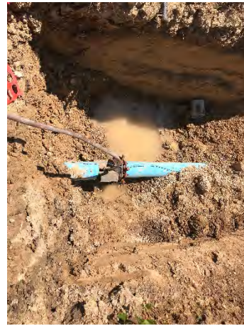
Picture of cap in place for forcemain pressure test.
