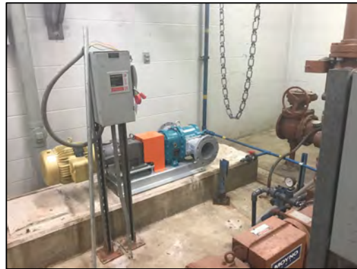
New rotary lobe pump being staged for install.
