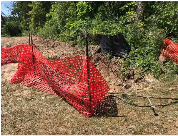
Cap location for forcemain pressure test performed on July 22 nd .
