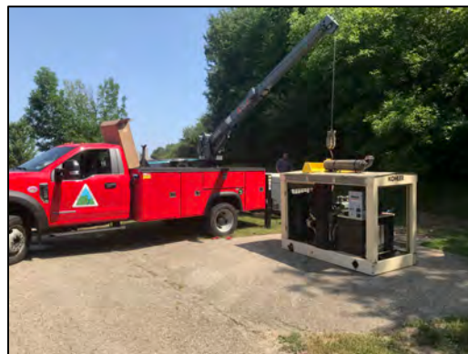
Old generator being removed.
