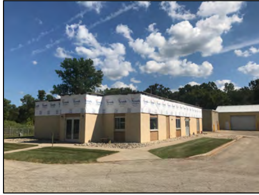
Moisture Barrier Tyvek Wrap over exposed CMU (cinderblock).
