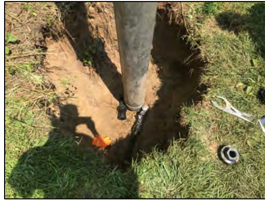
Hydro-excavation to reach break in low pressure force main.
