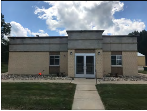
Mansard removed from Control Building.
