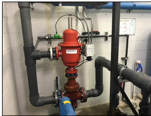
Strainer installed in NPW pump room.
