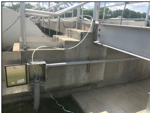
PVC conduit to house plastic chemical tube.
