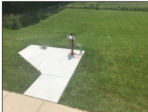
Actuator installed on new concrete pad.
