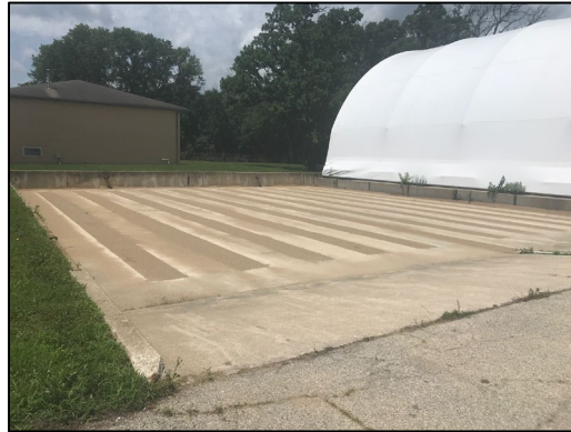
Fresh sand in drainage runners.
