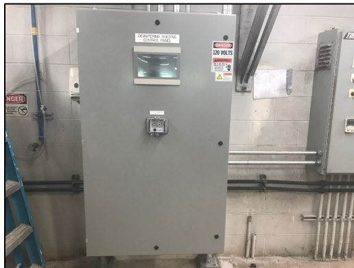
Dewatering Building SCADA panel.
