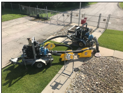
Bypass pumps staged upstream of headworks
