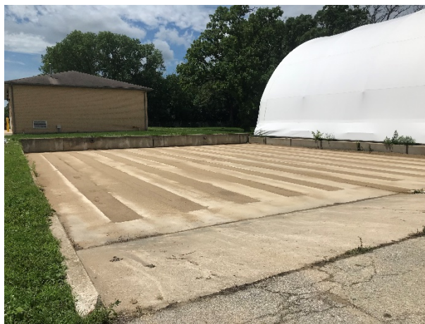
Drying beds after pavement removal and sand filler in runners.
